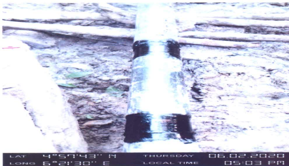
INCIDENT POINT AFTER REPAIR
